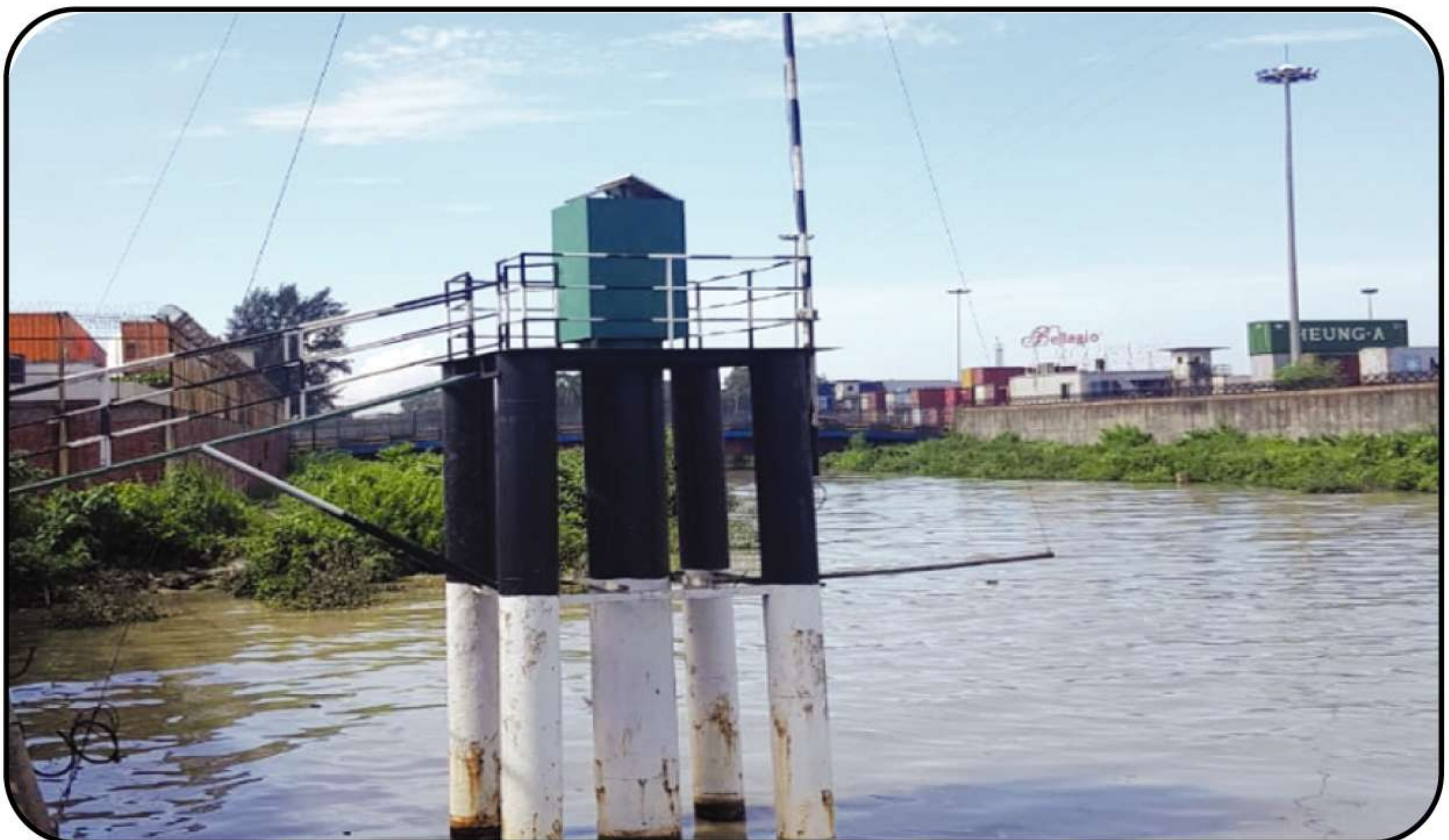
Auto Tide Gauge Station at Dock Office
