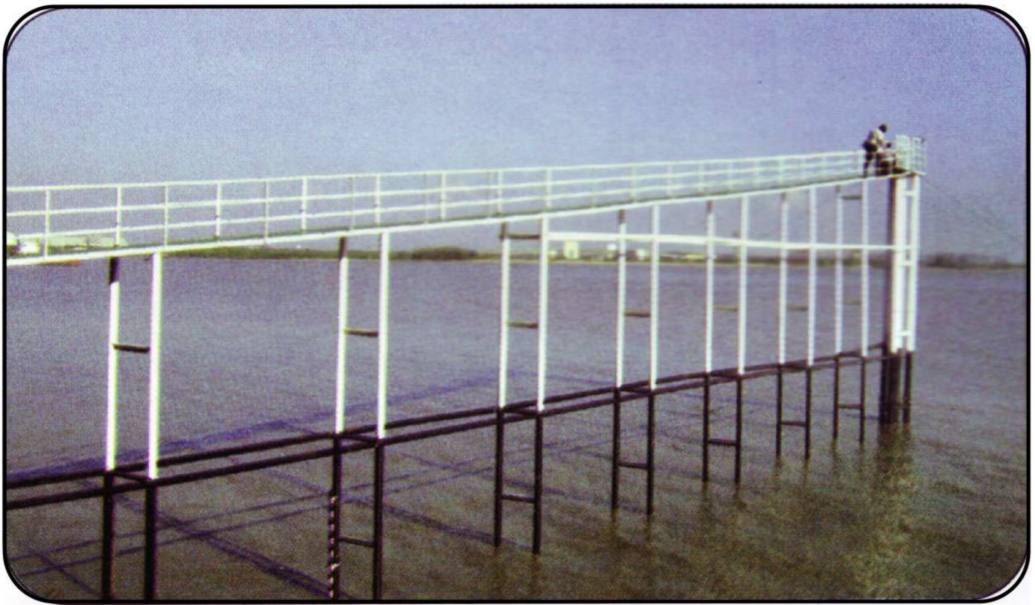
Auto Tide Gauge Station at Khal 18
